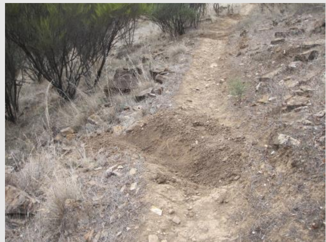
Three cross-track earth drains in a row
