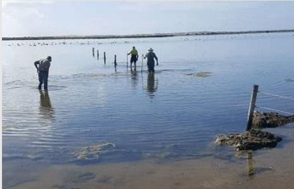
Dug out the old posts by hand (swans in the background)
