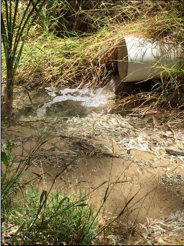
This photograph (taken on 11 January 2021) shows the amount of high saline/high chlorine water being discharged into Stonyfell Creek from the SA Water pipe.
