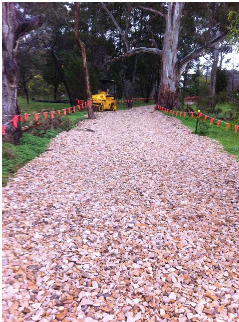
The temporary rubble track
