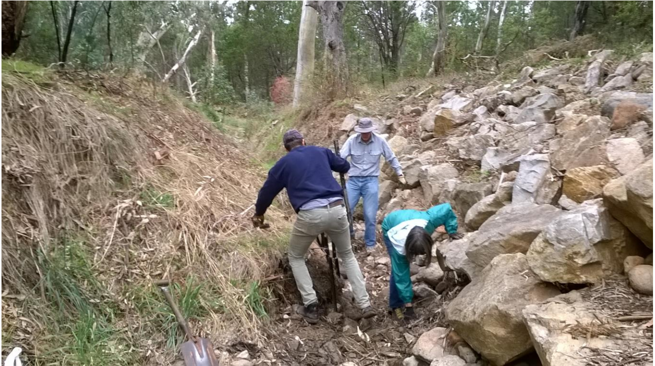
Stoneyfell Creek erosion control works – May 2017 working bee.
