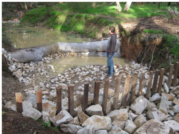
Pile drop weir (foreground) and log drop weir
