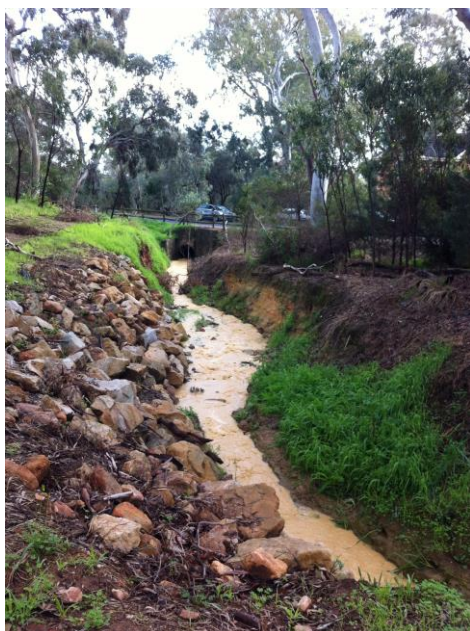
Completed Stage 1 erosion control works – June 2014
